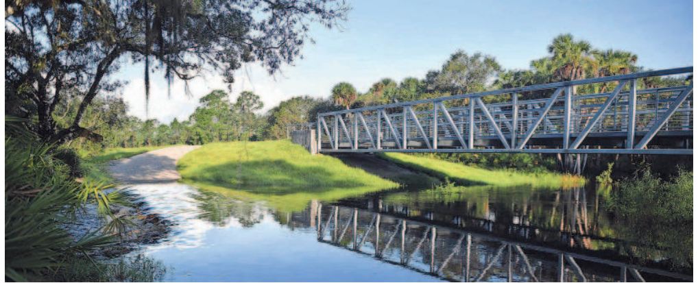
The bridge over Deer Prairie Creek is part of the North Port Connector of the Legacy Trail. The Gulf Coast Community Foundation has been a steadfast advocate for the Legacy Trail, providing more than $300,000 in financial support.
